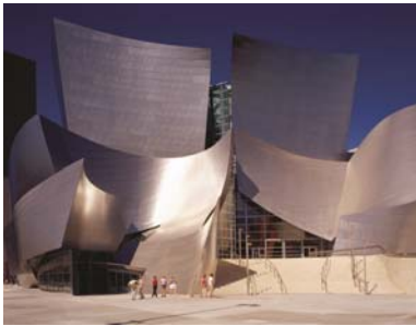
Courtesy of M. A. Mortenson Company
