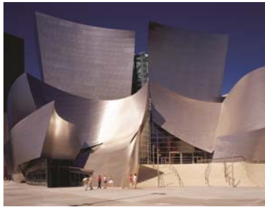
Courtesy of M. A. Mortenson Company
