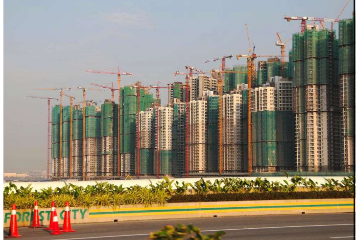
Johor's Forest City under construction [6]
