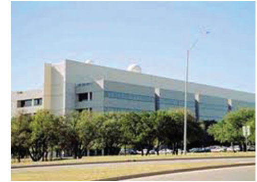
West Pickle Research (WPR) Building The University of Texas at Austin
